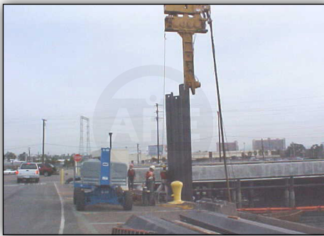
HYBRID EXTENSION CALLED THE CALIFORNIA STINGER FOR TIGHT WORKING DIMENSIONS.
